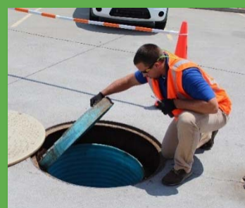
Inspecting a containment sump
